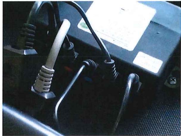
Lifting motor plug connected to control box.
